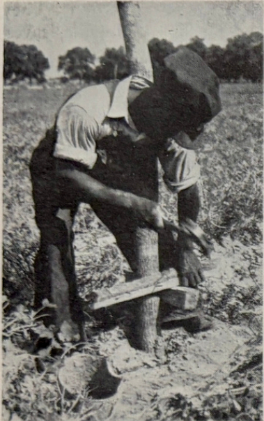
Place poles firmly in ground and nail two slats at right angles to the poles.
